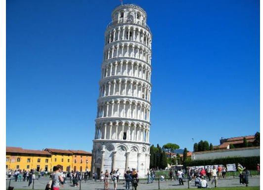
Leaning Tower of Pisa
